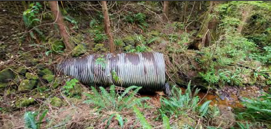
Photo 29. The Western Stream enters the southwest portion of the property from a large diameter culvert that crosses Peninsula Road. Showing culvert outlet.
