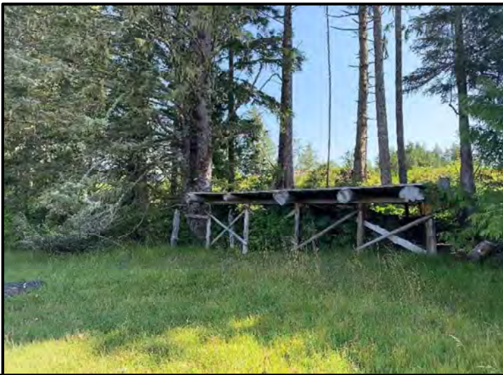
Photo 25. Narrow band of riparian trees along the northern tip of property. The wooden deck at shoreline built by previous owner without permit and should be removed.
