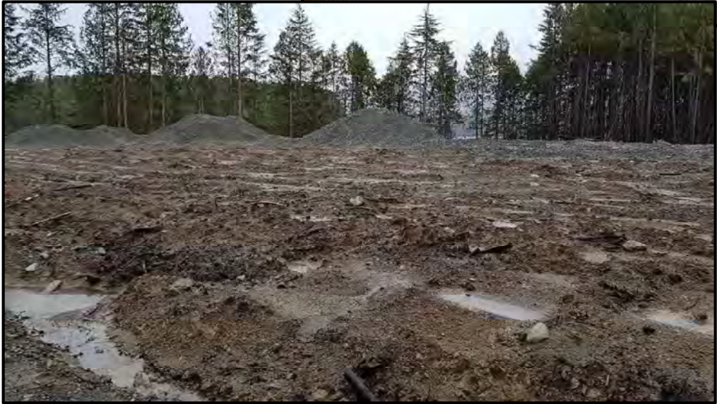
Photo 9: 2017 Image of cleared and grubbed section of site in northern half of property. Portion of foreshore buffer area cleared during tree removal.
